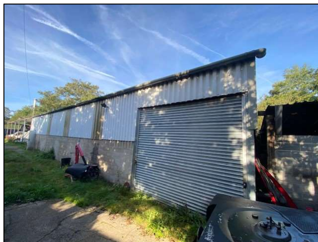
(Existing unit on the site)
